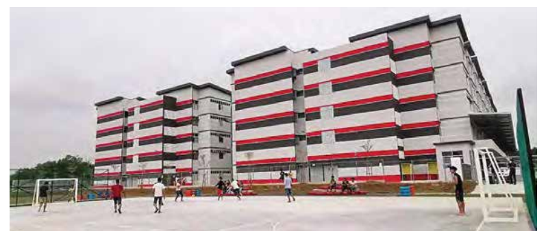
A worker's dormitory built to complement the industrial park, complete with a one-acre Sports Park.
